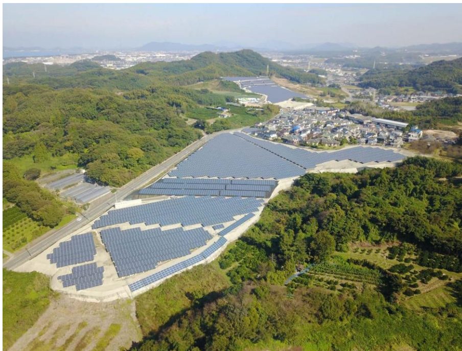
(Example) Solar power plant where jSEO provides O&M services
