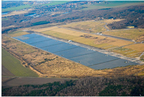
Construction status February 2008
