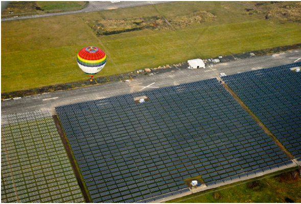
Construction status November 2007
